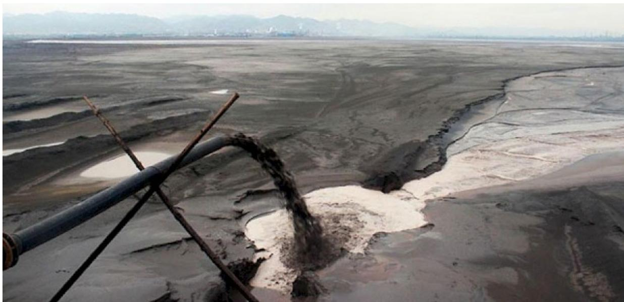
Figure 1 – Bayan Obo tailings dam - note the plant in the rear
