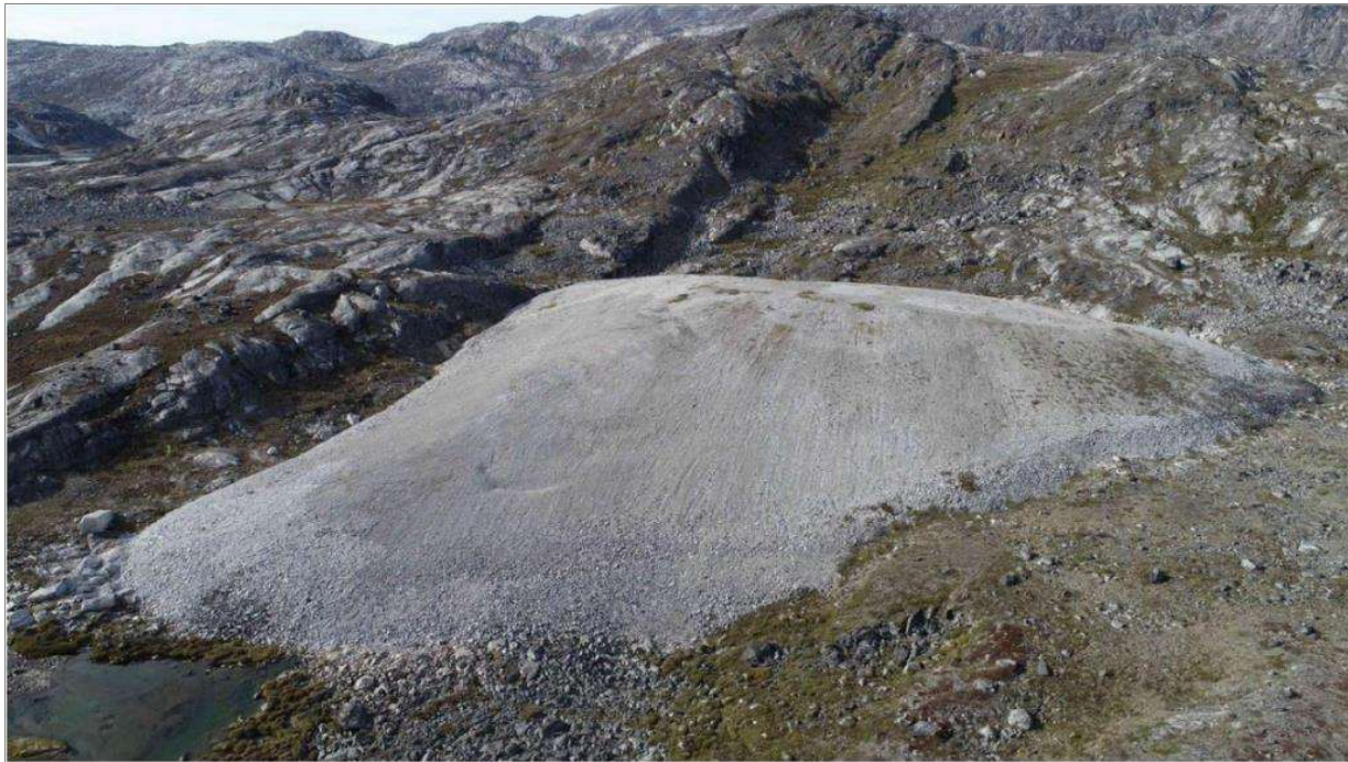
Figure 80: Example of a large blast rock deposition site following a hydropower project. The potential project TSF will be several times larger.
