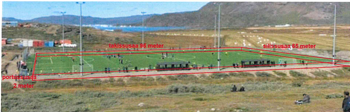
Asseq 4. Kuannersuarni qaartitsinerit tamaasa qaartinneqartussaq assilianngorlugu: Narsap Arsaattarfiata angeqataa ammallu = 96 \text{ m} \times 65 \text{ m} \times 2 \text{ meter} .
